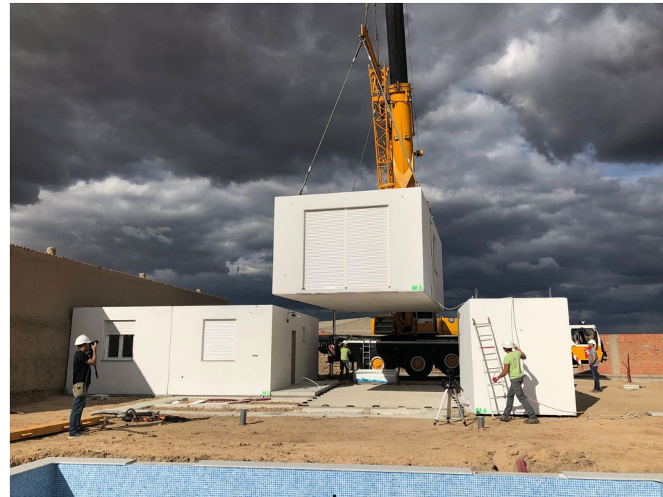
3D: módulos completos (<95% obra off-site)
