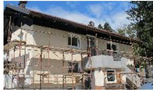
Case 6: Monitoring solution of complete energy renovated single-family houses, Slovenia
