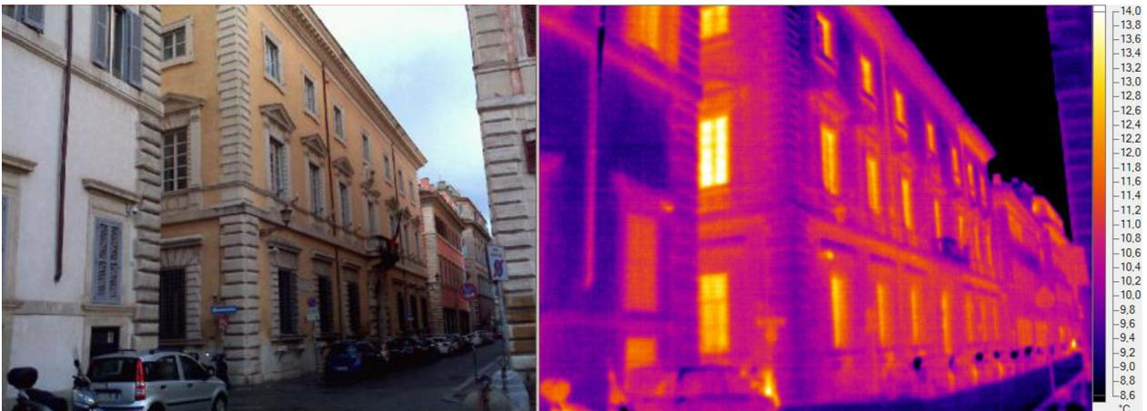
Fig. 7. Comparison between the photography and the termographic image of the main façade of Palazzo Maffei-Borghese, Rome.
