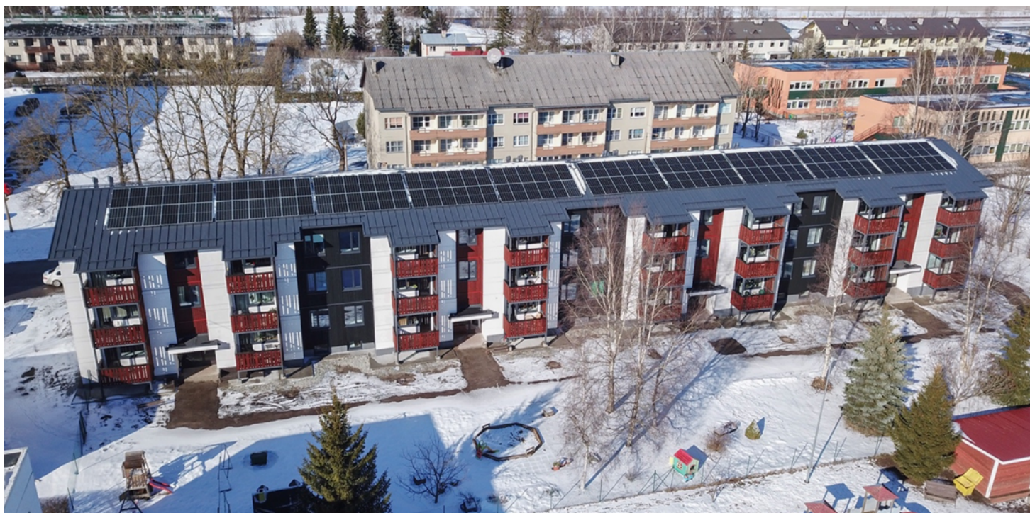
Figure 1. Estonian pilot: residential building located in Saue. General view after the deep renovation intervention based on the implementation of a circular strategy: extension of net area by closing balconies for enlarged living spaces and implementing façade additions for new balconies; energy refurbishment of the envelope through prefabricated modules with reused and recycled materials and bio-based material, and building integrated renewable energy technologies. (Source: TalTech and TIMBECO, 2023)
